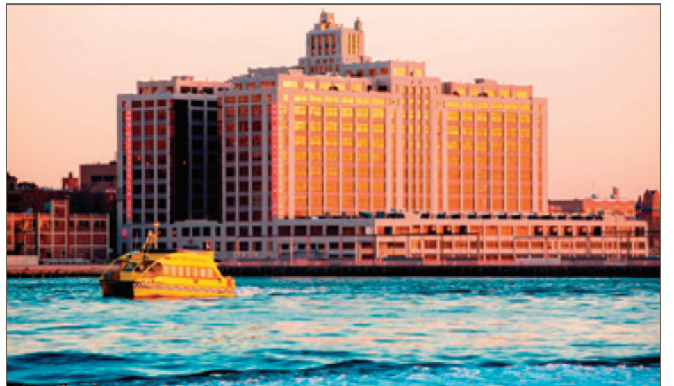
THIS IMAGE SHOWS ONE BROOKLYN BRIDGE PARK AS SEEN FROM THE WATER. The developer of the luxury condo conversion at the south end of Brooklyn Bridge Park has hired a new leasing agent to find commercial tenants for 68,000 square feet of vacant retail space. See Eye on Real Estate, Pages 1-2INB.
