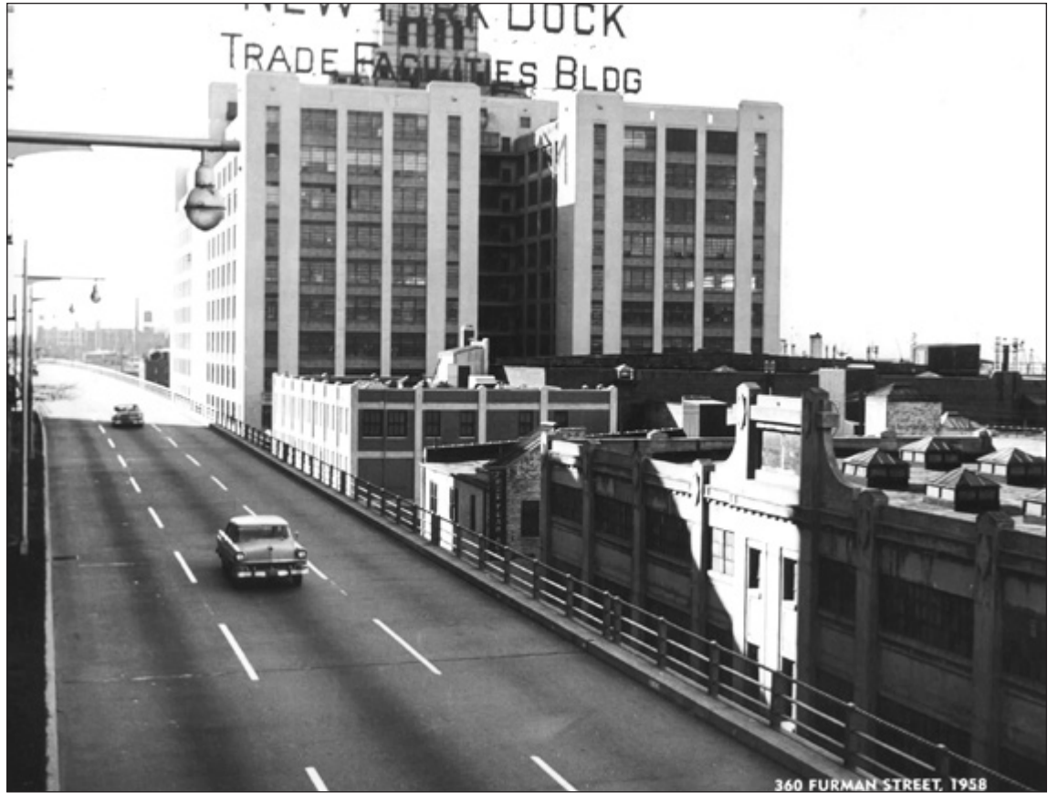
This 1950s photo shows One Brooklyn Bridge Park when it was an industrial building, before the Jehovah's Witnesses owned it. Eagle file photo
