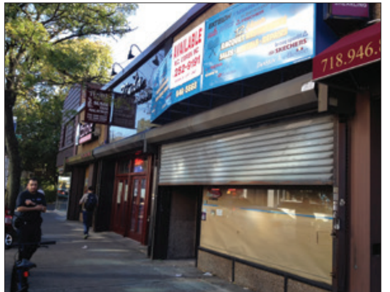
This Sandy-struck Sheepshead Bay Road storefront, formerly occupied by Bay Sports, is getting a new tenant. Photo by Lore Croghan
