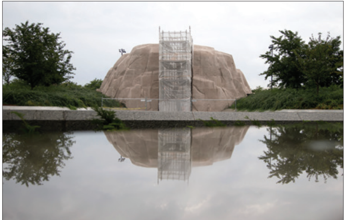
KING MEMORIAL: Scaffolding rises from the Martin Luther King Jr. Memorial as it is reflected in a puddle on a rainy Tuesday in Washington. Work to refinish part of the Martin Luther King Jr. Memorial, where a disputed inscription was recently removed, might not be done until after the 50th anniversary of the March on Washington. AP Photos
