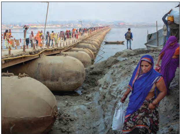
A pontoon bridge traditionally uses anchored floats to create a continuous passageway for pedestrians and vehicles. AP Photo/Rajesh Kumar Singh
